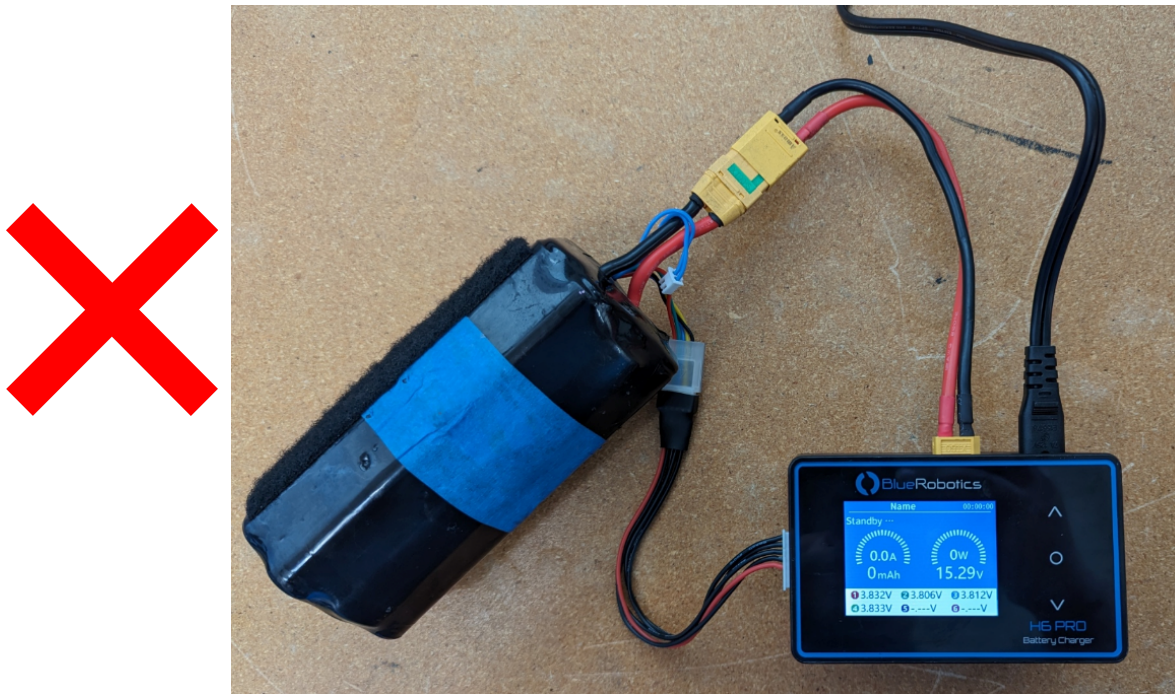
Figure 2. Incorrect battery connection. The battery is connected to the DC IN port. This will lead to fire hazard.
